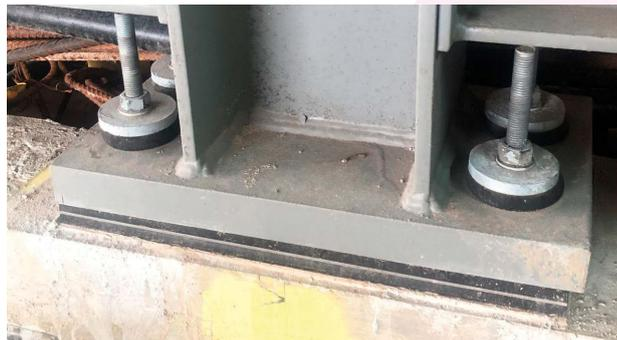
Farrat Hybrid Bearings used to isolate the steelwork to the new rooftop extension
