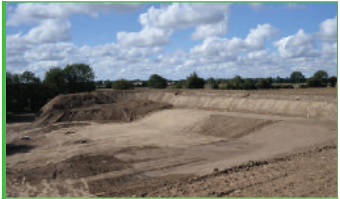
Figure 11. Construction of soil banking
