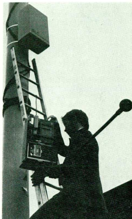
Fixing a BLEEP to a flag-pole — now usually done by means of a 'Skyraker' platform
