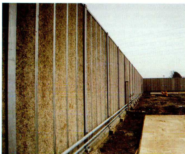
External noise barrier constructed from 100 mm thick, 4m long WOODCELIP slabs.
