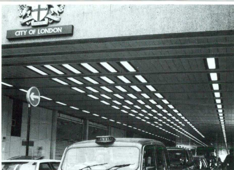
Tufsound Acoustic panelling used at Beech Street road tunnel
