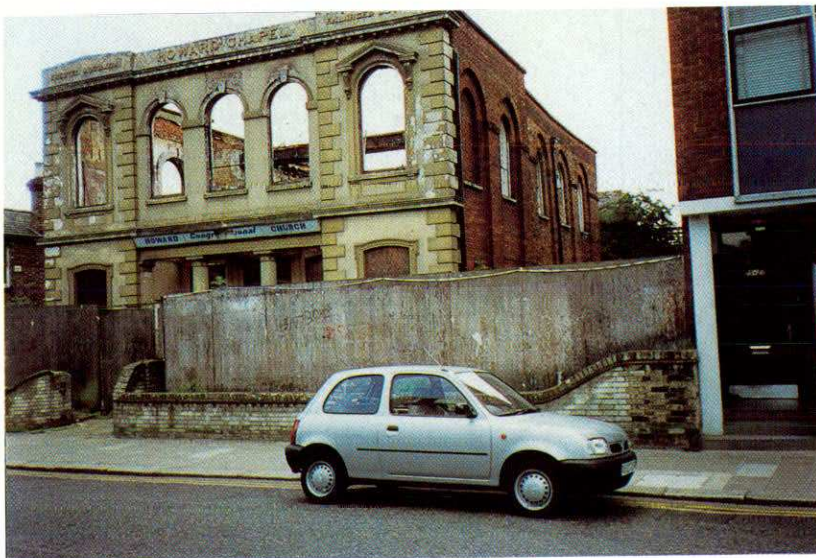
Fig. 1. Listed façade of the chapel
