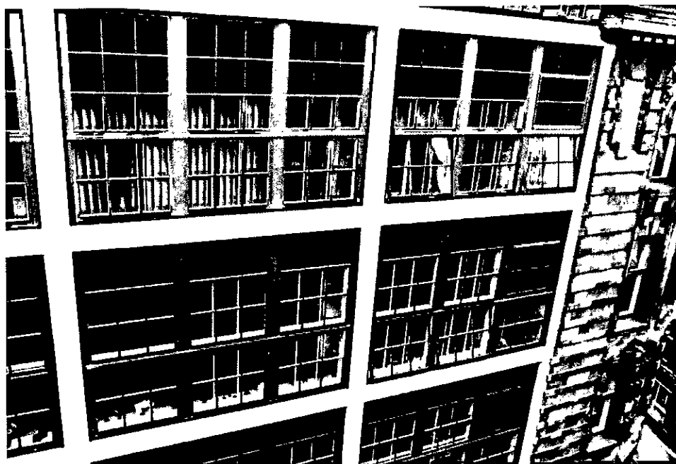
Flanking transmission between adjacent apartments can be a particular problem on refurbishment projects
