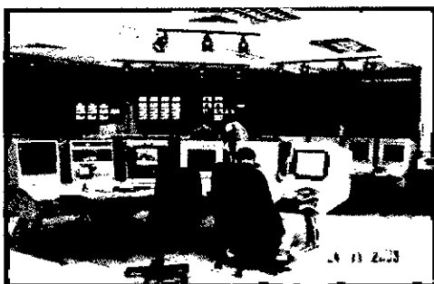
4 The master control room
