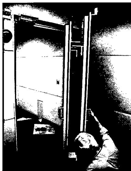
9 Space constraints necessitated a compromise 'piggyback' door arrangement
