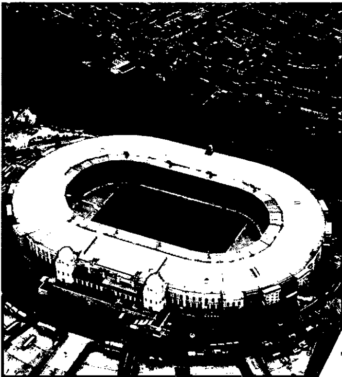
The old Wembley stadium was fitted out with a sound system of professional grade with digital signal processing and fibre optic signal distribution
