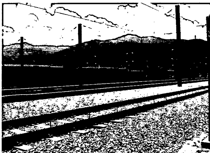
'Noise was considered from all possible viewpoints uniting track bed, rolling stock and station design'
