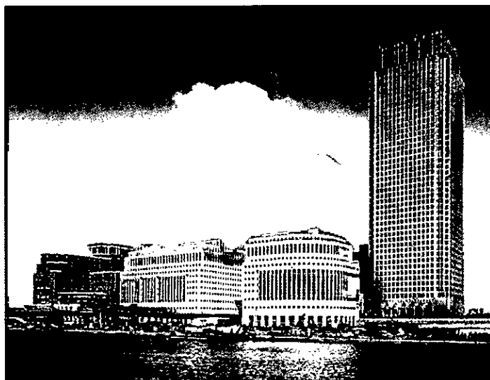
The consultants were asked to help a client in Canary Wharf to find the real source of the failure of the Voice Alarm (VA) system to broadcast an intelligible live announcement
