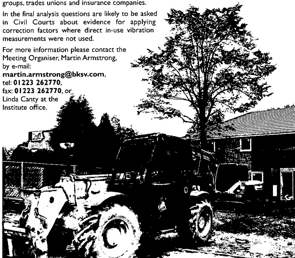
Whole body vibration as experienced by plant operators is covered by the Control of Vibration at Work Regulations
