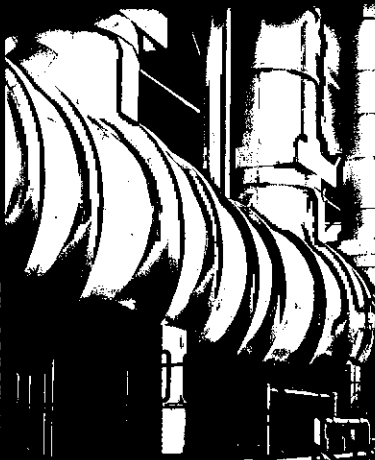
CCGT Power Station, Uskmouth Bespoke Acoustic Lagging System
