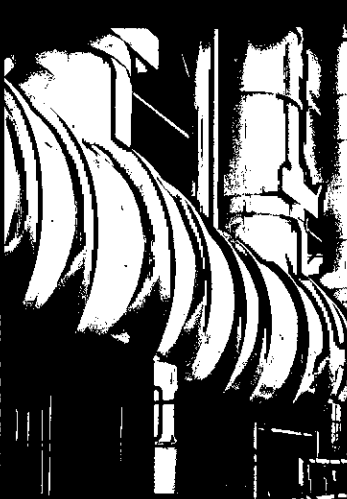
CCGT Power Station, Uskmouth Bespoke Acoustic Lagging System
