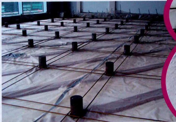
Construction phases of a spring floating floor
