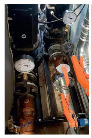
The GSHP system distributes hot water directly through the building's radiators and indirectly provides the building's domestic hot water via a heat exchanger. The system comprises:
