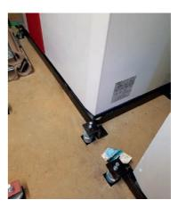
Above: Figure 5 GSHPs on isolated frames (fitted whilst the plant remained operational)
