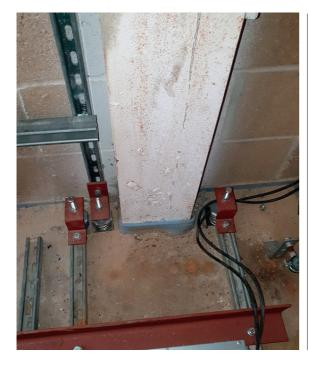
Left: Figure 9 Strut channel decoupled from wall and floor with isolated support brackets
