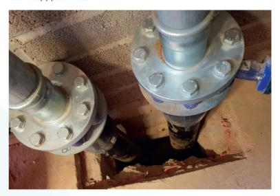
Above: Figure 12 Ground loop pipes broken out
