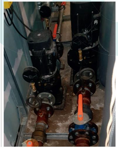
Figure 1 Ground loop pumps on resilient pads
