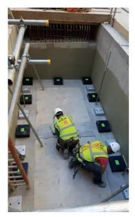
the adjacent tube line and road would have re-radiated as undesirable noise levels within the building, a 25dB(A) criteria applied. The project was challenging in that the isolation line had to be accommodated with minimal disruption to the existing design.
