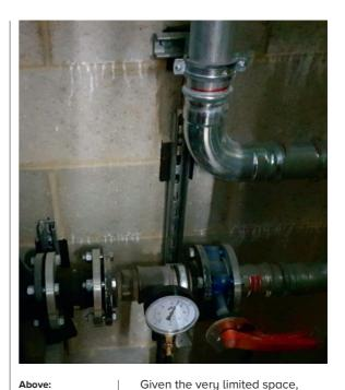
Above: Figure 7 Strut Channel bolted to wall with resilient pads
