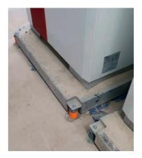
Above: Figure 4 GSHPs on inertia bases. The springs provide vibration isolation, but the concrete is unnecessary
