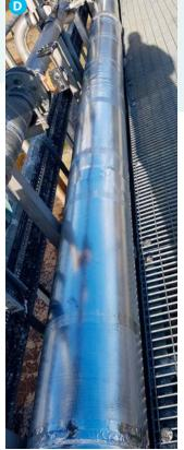
Due to the variable nature of operation of the blowers it is not practicable to directly compare sound level measurements before and after treatment to assess the effectiveness of the cladding system. A similar arrangement has previously been used to reduce noise radiated by the body of a generator exhaust silencer. Figure 8 shows the sound intensity level emitted by the exhaust silencer body before and after being clad in the frequencies of interest.
