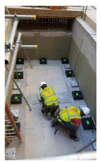
the adjacent tube line and road would have re-radiated as undesirable noise levels within the building, a 25dB(A) criteria applied. The project was challenging in that the isolation line had to be accommodated with minimal disruption to the existing design.
