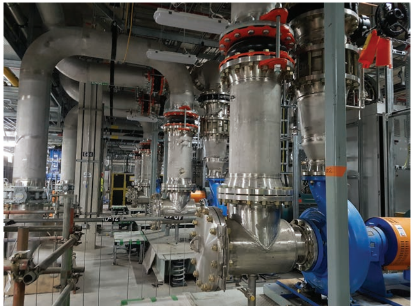
► Inertia bases, flexible connectors and pipe isolation system for Intel Corporation, Dublin.
