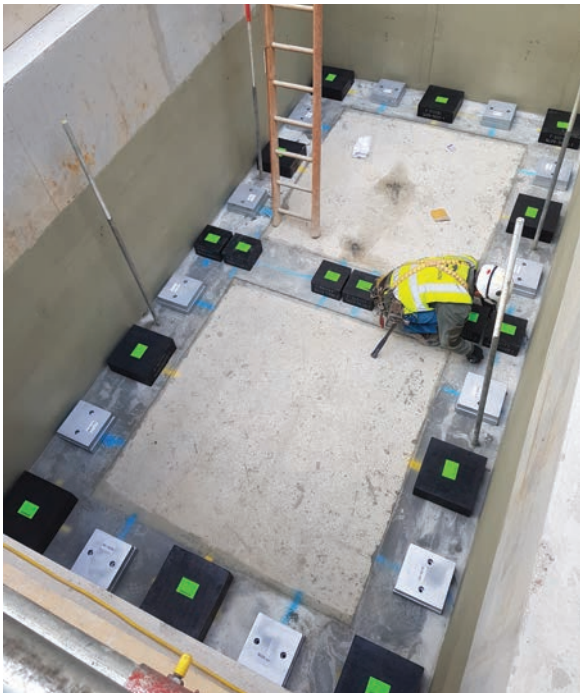
► Inertia bases, flexible connectors and pipe isolation system for Intel Corporation, Dublin.
