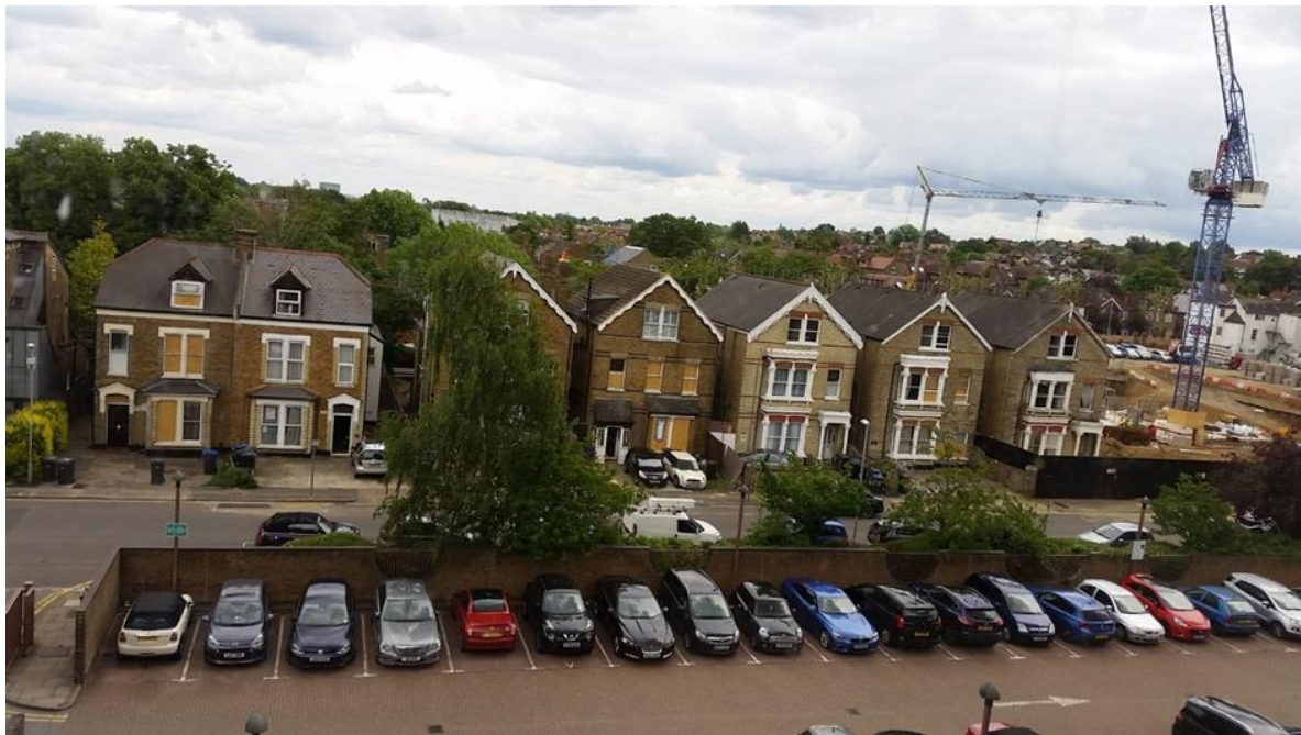
Figure 2 : Photograph of the area of the bomb site, taken a few days after the detonation, showing boarded-up windows which had been damaged as a consequence of the bomb's detonation on houses on Fasset Road, immediately to the North of the bomb's position (close to the blue crane on the right of the photograph). The pattern of damaged and undamaged windows is discussed below. Very few windows in houses to the South of the bomb's position were damaged, and those which were damaged on that side were all in direct "line of sight" from the point of explosion.
