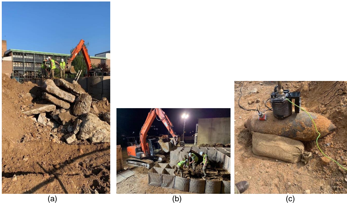
Figure 4 : Some photographs, courtesy of the Royal Engineers of Carver Barracks, showing aspects of the site prior to their controlled detonation of the bomb. From left to right : (a) Engineers filling sandbags around the bomb. Kingston University's Sopwith building can be seen in the background. The rubble in the front of the image is left over from the demolition of the buildings of the hotel located there until a few weeks before the photograph was taken, and is not directly related to the bomb explosion. (b) later in the same operation. Sand bags can be observed to be in place on three sides of the bomb at this point. (c) A close-up of the bomb and the detonator which the Engineers had attached to it. Part of a soldier's booted foot can be seen in the bottom left of this photograph, to provide a sense of scale.
