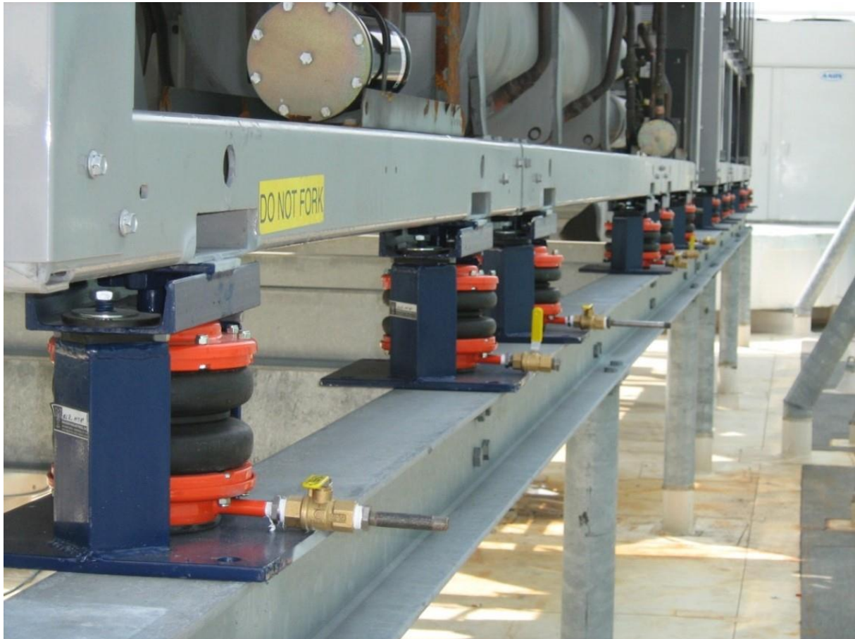
Figure 2 – Example of air spring supported equipment
