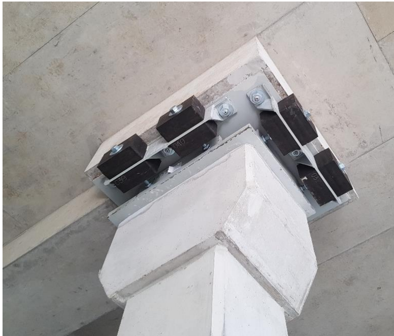
Figure 4: Column head assembly with bolt-on lateral braces (gravity-loaded bearing not visible)
