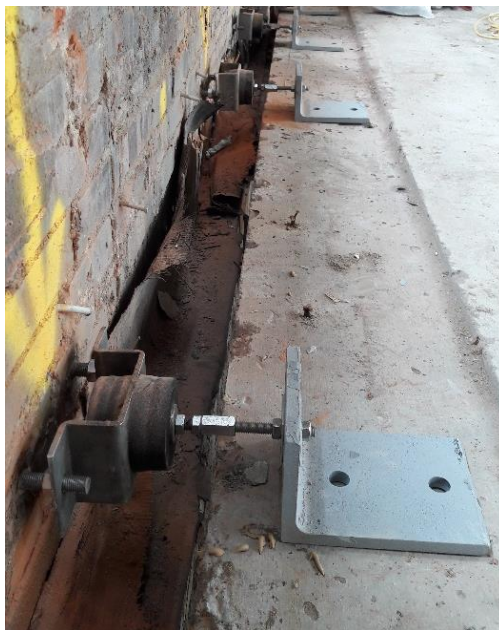
Figure 5: Uni-directional facade braces designed to a precise spring rate
