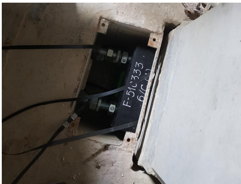
Figure 3: Core lateral restraint bearing with hardware to apply a prescribed compression
