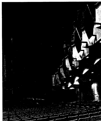
Figure 5. Zone 2 balcony fascia reflectors are seen in the foreground. Note how they progressively move toward the centre-line of the room. The Zone 1 proscenium reflectors are seen in the background.
