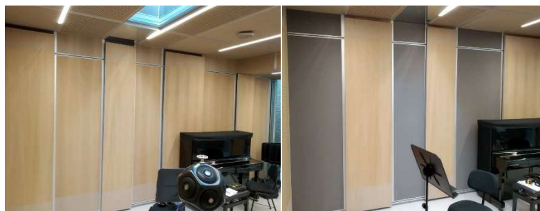
Figure 15 Two different settings of sliding wall panels in rehearsal studio (reflective (left) and absorptive (right))
