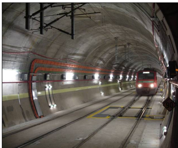
Figure 2: Multimodal platform with embedded slab track in Rossio tunnel
