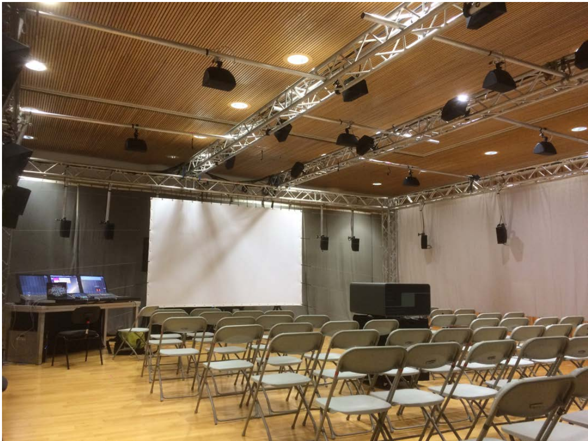
Figure 4: Temporary installed Dolby Atmos / IOSONO / AFC3 system at Berklee College of Music
