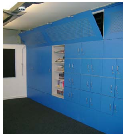
Pic 18. Vents within classroom – Vent open within left hand side image – School G
