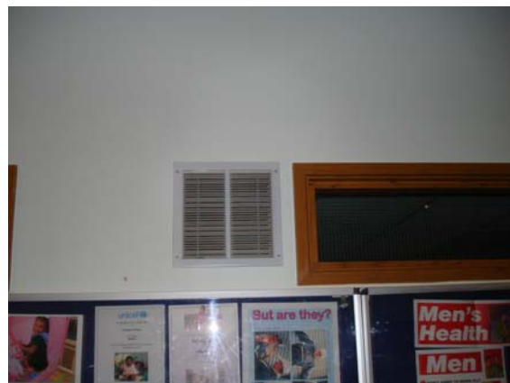
Pic 13. Corridor walls including un-attenuated vent – School E
