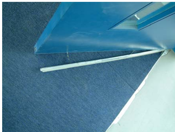
Pic2. Drop seal pulled out from under door
