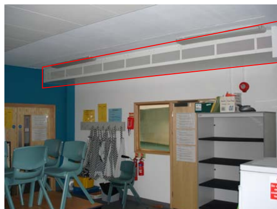
Pic 19. Attenuator ventilator within classroom Ground Floor – School H
