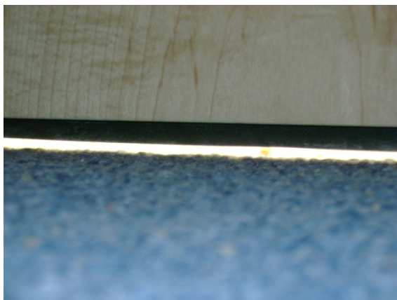
Pic 1. Drop seal falling short of the floor finish
