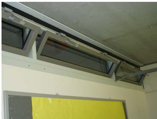
Pic 10. Un-attenuated vent to central Atrium – School D
