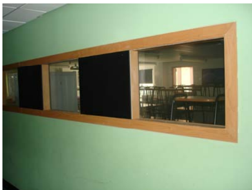
Pic 9. Poor detailing around a Vision Panel
