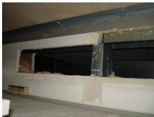
Pic 9. Plasterboard missing at the top of partitions
