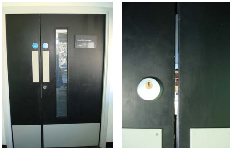
Pic 5. Large gap between double and leaf & a half doors – a very common fault
