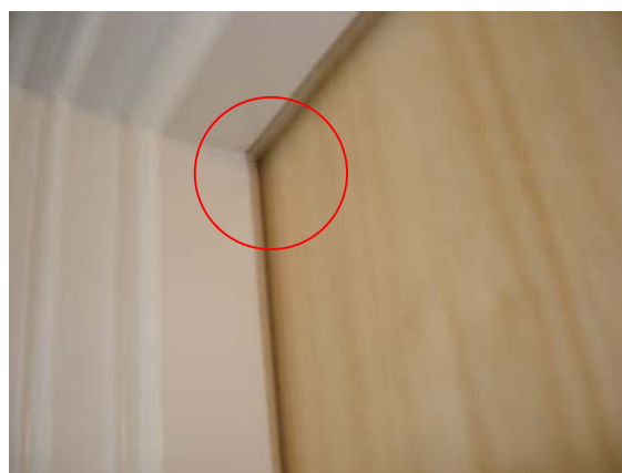
Pic 7. Gap – Door head-leading edge bending away from the door rebate, A common fault
