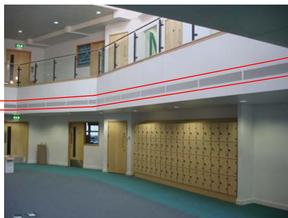
Pic 19. Attenuator ventilator within classroom Ground Floor – School H
