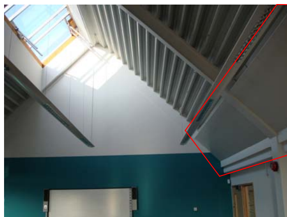
Pic 20. Attenuator ventilator within Classroom First Floor – School H
