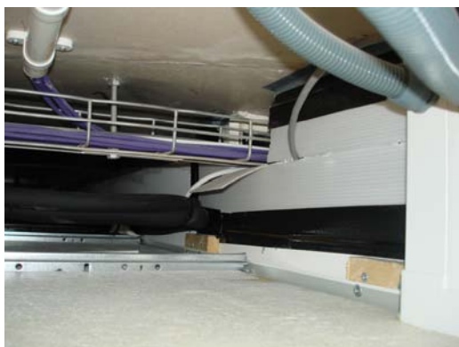
Pic 8. Poorly sealed service penetration
