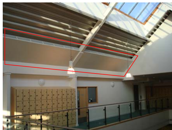
Pic 20. Attenuator ventilator within Classroom First Floor – School H
