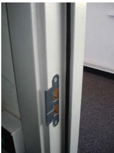
Pic 4. Door locks cutting through wiper seals – correct detail on the right
