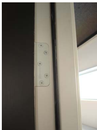
Pic 3. Hinges cutting through wiper seals – correct detail on the right
