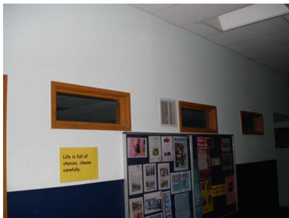
Pic 13. Corridor walls including un-attenuated vent – School E
