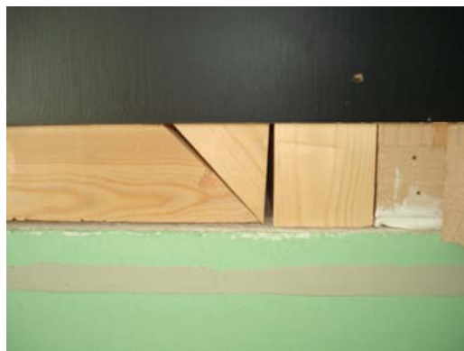
Pic 9. Poor detailing around a Vision Panel
