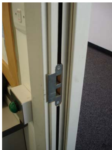
Pic 4. Door locks cutting through wiper seals – correct detail on the right
