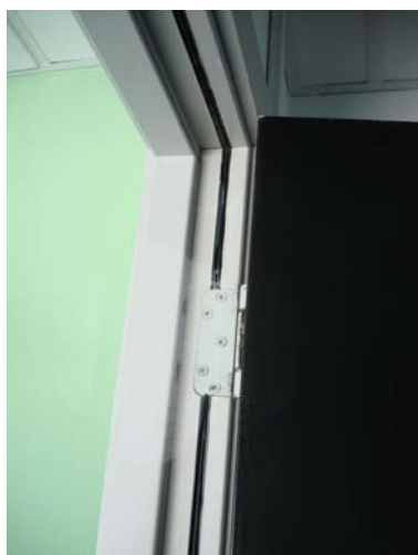
Pic 3. Hinges cutting through wiper seals – correct detail on the right
