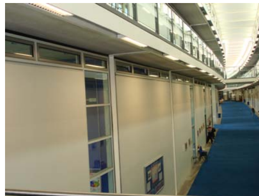
Pic 10. Un-attenuated vent to central Atrium – School D
