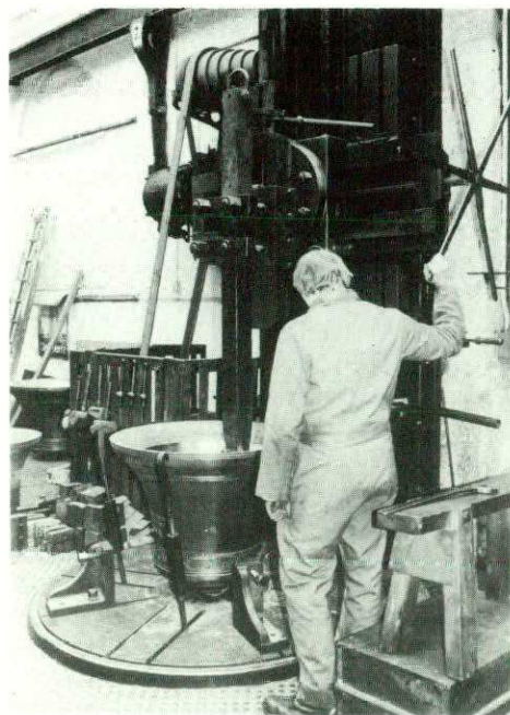
Figure 3 Bell tuning at Taylor's Bell Foundry, Loughborough
