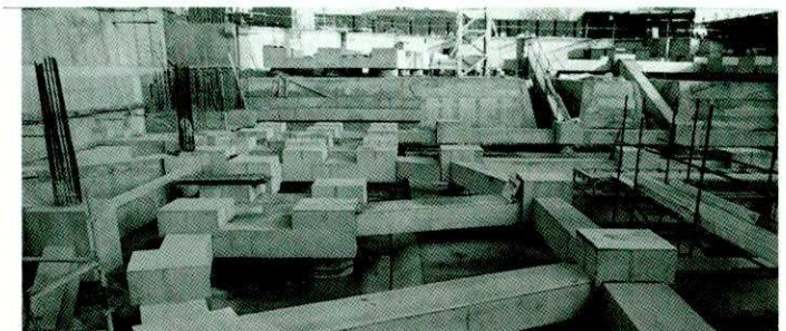
Fig. 5. Undercroft showing the beams.
