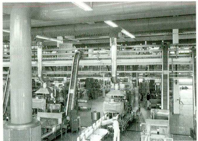
Ecophon Hygiene ceiling in a Swedish Dairy
