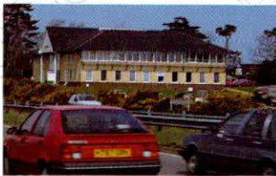
Noise from traffic at Brightwell Court, adjacent to the busy A12 at Martlesham, was controlled using MODUL windows
