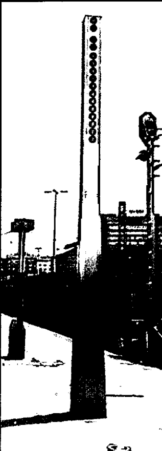
Budapest Station, Hungary - one system provides sufficient coverage for a long platform.
