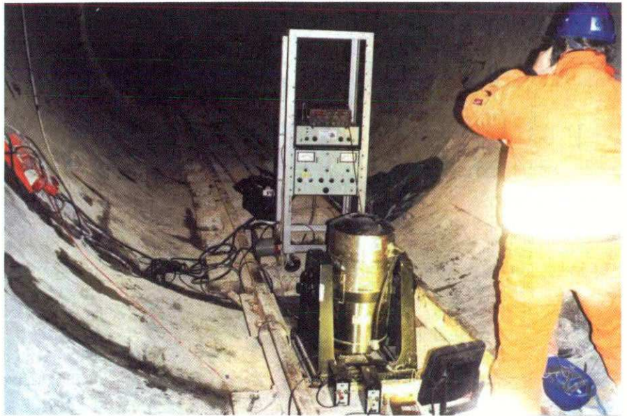
Fig. 2. The vibration exciting equipment
