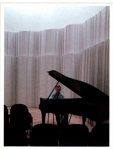
Fig. 4. View of diffusing wall in completed hall
