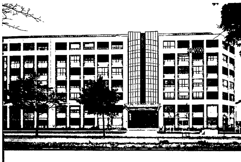
Figure 2: A typical base-isolated building in the form of a multi-storey office (courtesy of GERB Schwingungsisolierungen GmbH & Co, Germany). The entire building is isolated from its foundation by spring bearings located in the basement
