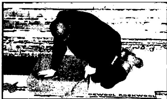
FIGURE 02 Rockwool Hardrock being laid on vapour control layer
