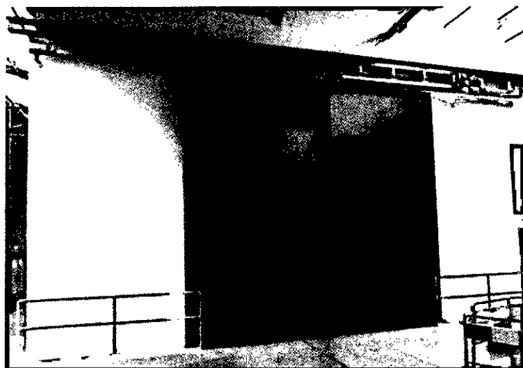
5m x 5m bi-parting horizontal acoustic door
