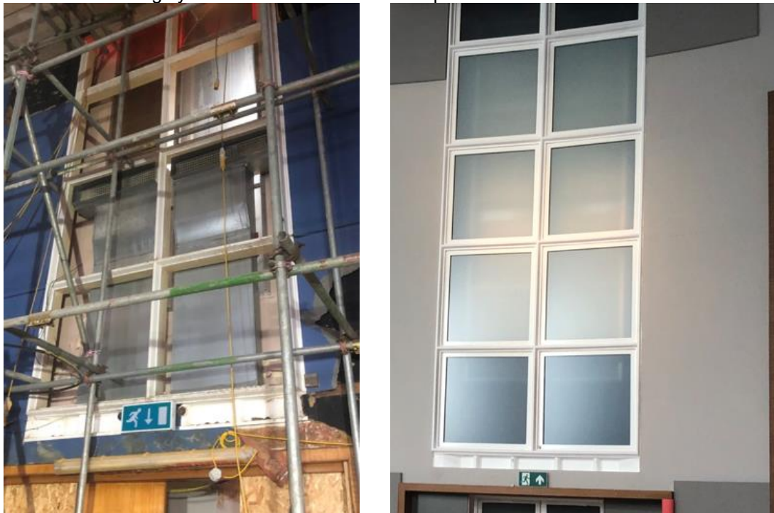
Figure 7 Glazed elements within separating walls (existing left, refurbished right)
