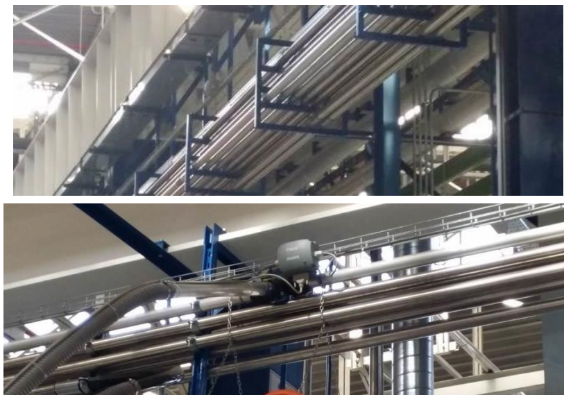
Figure 3: Large and small resin distribution networks
