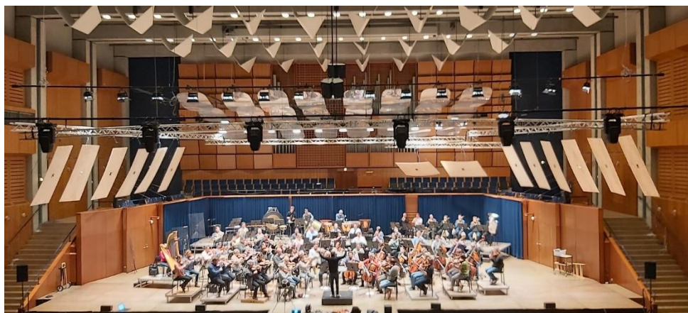
Fig. 6 Tilted reflectors installed for the last day of testing, 23rd February
