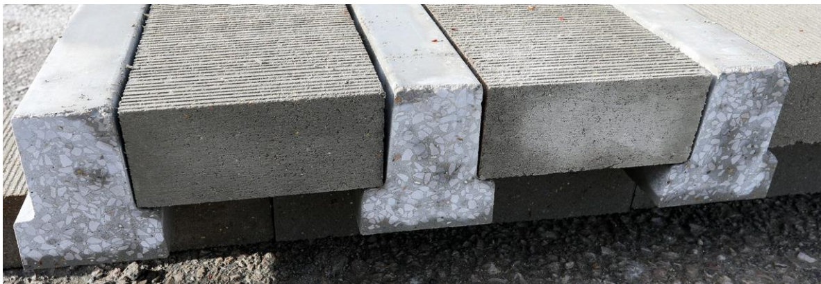
Figure 6 Typical beam and block floor
