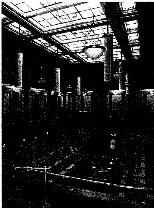
Figure 3: Six "Kiwi-tubes" in situ at 6 metres height
