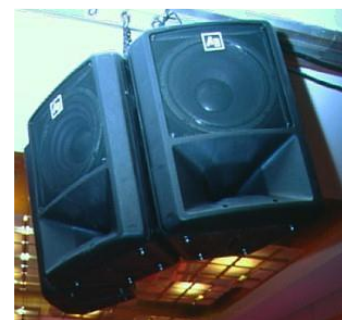
Figure 2. Typical two-element cluster
