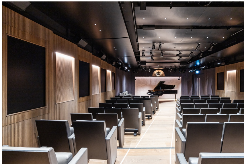
Figure 1: Photo of Bechstein Hall showing curved ceiling and soffit panels and vertically inclined wall segments. Active acoustics system loudspeakers can be seen above the side wall panelling and between the ceiling panels.
