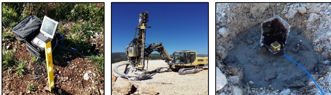
Fig. 2 : correct alignment control (left figure), puncher machine (central figure) and the iron spike immobilized with the cement (right figure)
