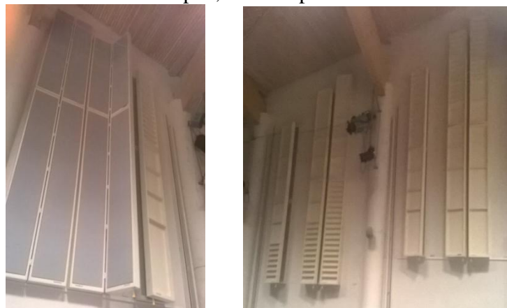
Figure 1: Variable absorption elements (“Flip-Flops”) in the Topelius hall in Sibbo, Finland
