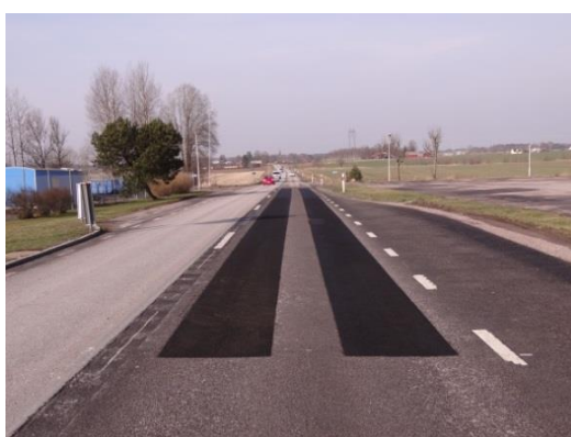
Figure 5 The PERS track in Sjögestad in April 2016 (after two winters, left hand side) and results of noise measurements with the CPX at 80 km/h on some PERSUADE PERS test tracks, compared to references used in some countries. The Sjögestad test track with PERS panels on semiflexible is indicated with “PERS-SE2-HET2”
