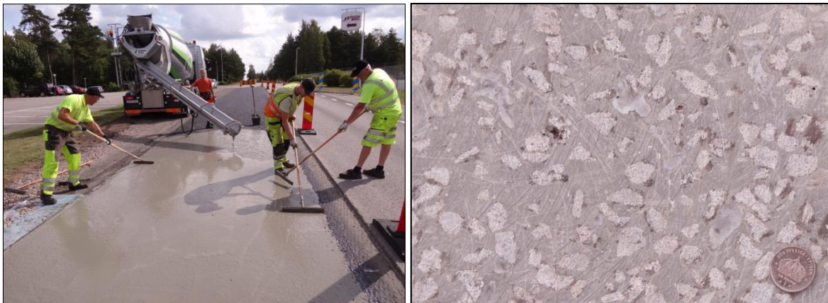
Figure 3 Filling of the voids of the porous asphalt with the fine-graded cement slurry and the polished surface of the under layer
