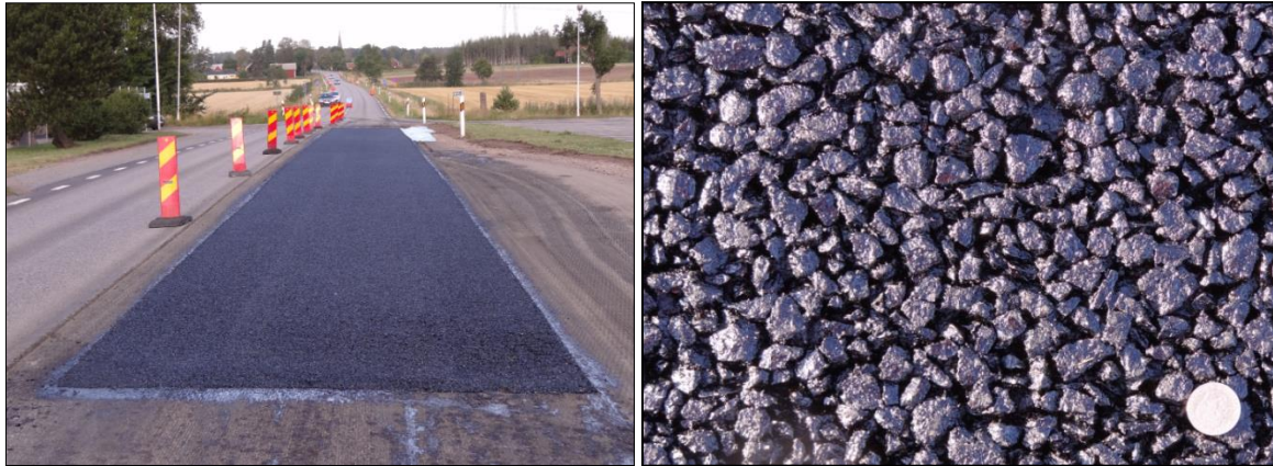
Figure 2 Porous asphalt 0/16 under layer (coin on the right hand side has a diameter of 25 mm)
