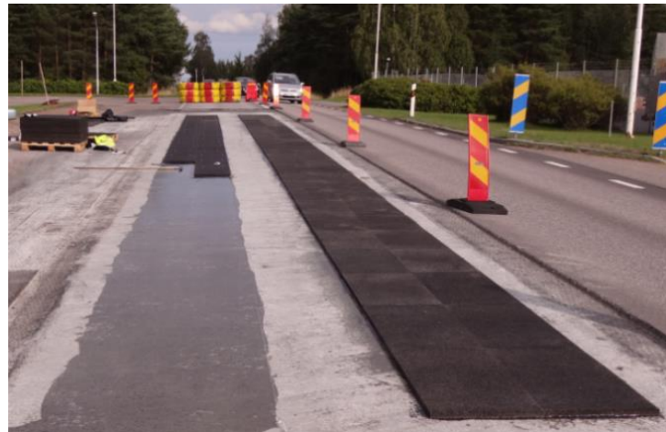
Figure 4 The PERS track in Sjögestad (two strips in wheel tracks) under construction
