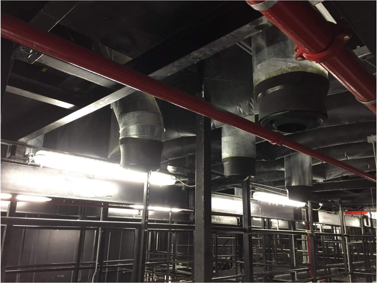
Figure 5: Inflatable low frequency absorbers installed above gantry level
