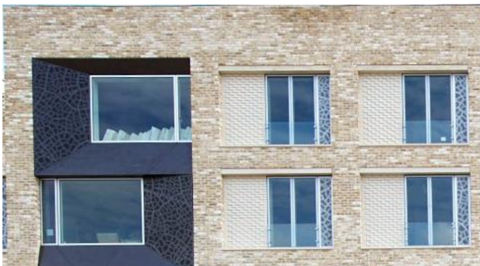
Figure 4: Lot 5 façade showing perforated panels adjacent to windows
