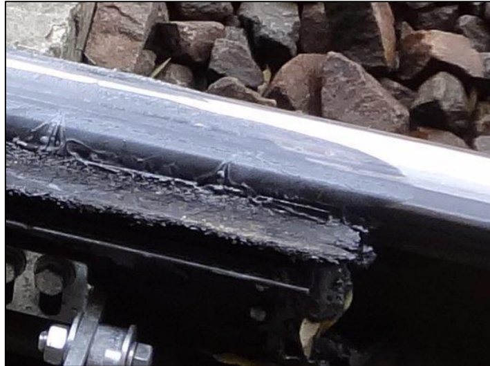
Figure 6: Rail lubrication equipment 1
