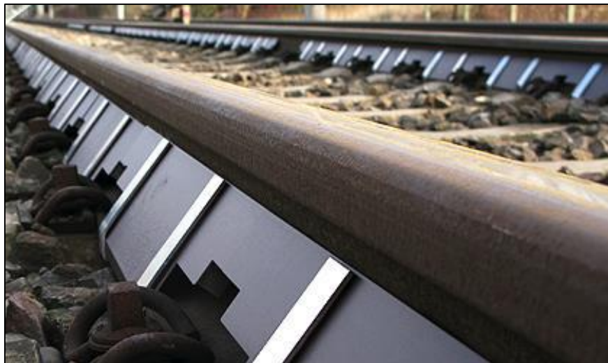
Figure 5: Rail web shielding 5
