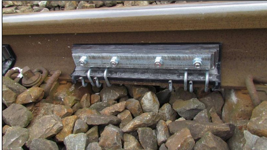
Figure 4: Rail web damper 1
