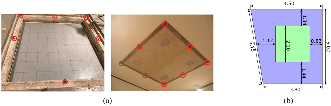
Figure 4: The concrete floor between two transmission rooms: (a) the upper and lower surface of the suspended concrete floor. The bolts are indicated by circles. (b) the top view of the full floor. The dimensions are in meter.
