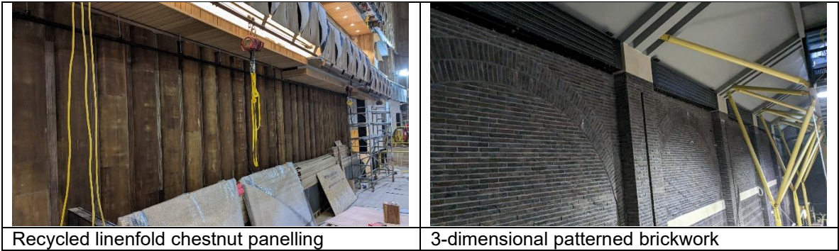
Figure 5: Traditional finishes - timber on solid backing and patterned brick with stiff supports
