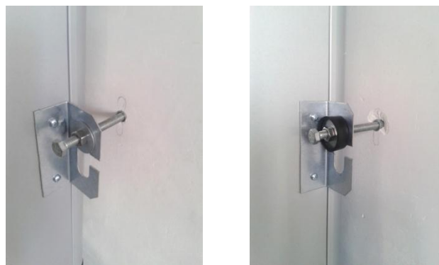
Figure 1: Rigid mounting (left) and mounting with vibration isolator (right).
