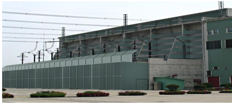
Fig.2 The sound barrier for converter transform
