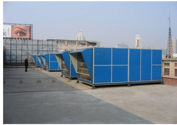
Fig.4 Box-in for the fan in main transform room
