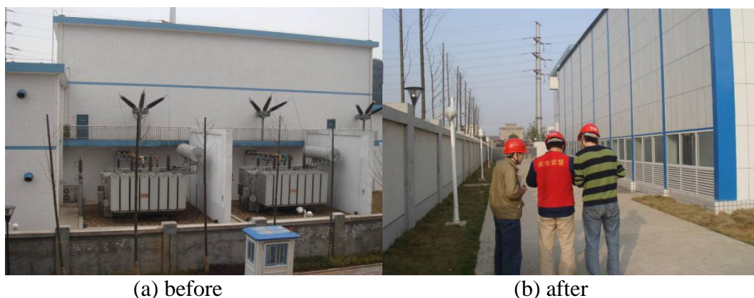
Fig.1 The sound barrier for outdoor transform
