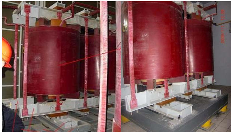
(a) before (b) after Fig.9 A vibration isolation device for the indoor reactor
