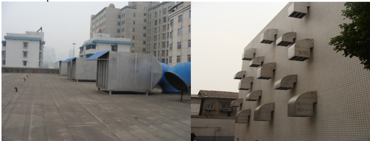
Fig.5 The muffler for fans in main transform room Fig.6 The muffler for fans for the capacitor room
