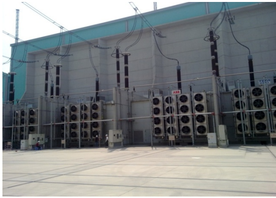
Fig.3 Box-in for converter transformer
