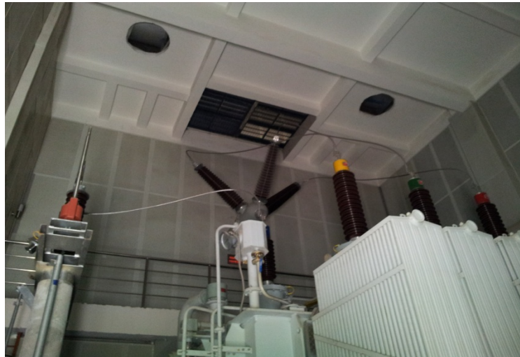
Fig.8 The microperforated panel for main transformer chamber
