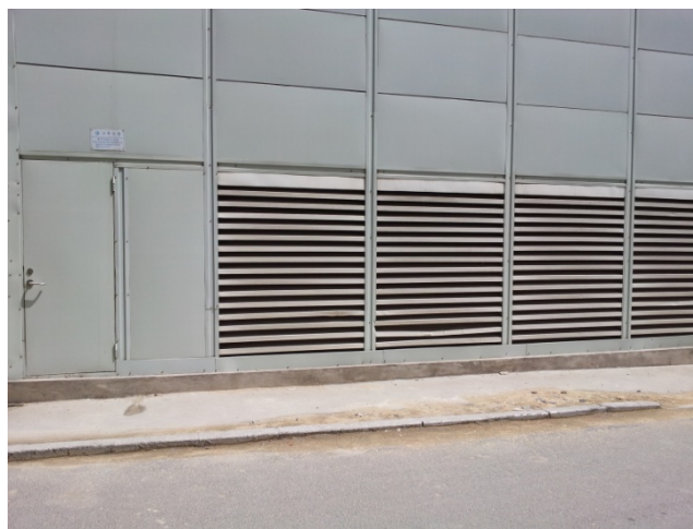
Fig.7 The fixed sound proof door with a small-sized maintenance door
